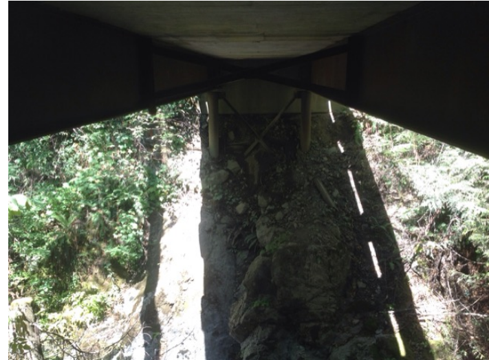
Left Bank Abutment when facing downstream
