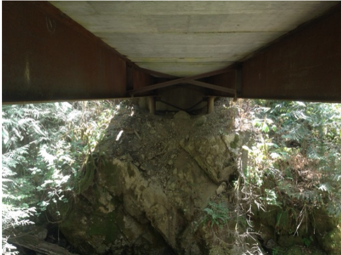
Right Bank Abutment when facing downstream
